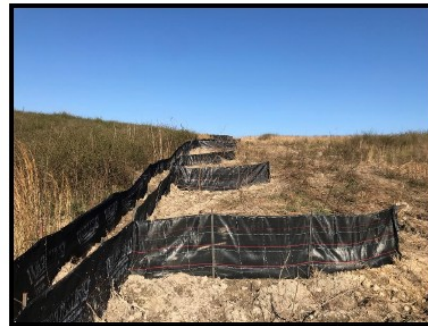
Image 3 - Sd1-S – Silt Fence Type Sensitive- J-Hooks for Slope on CE 1.04
