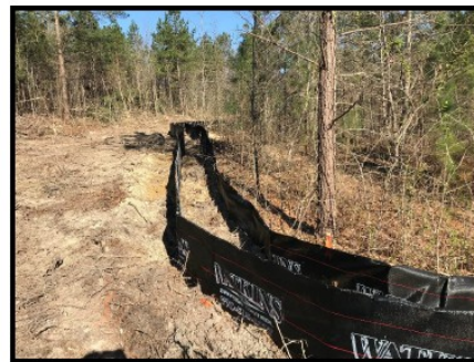
Image 4 - Sd1-S – Silt Fence Type Sensitive- Double Row – Borrow Pit
